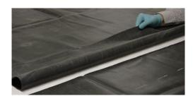
2. Fold back the top liner (you can use a small amount of the QuickPrime Plus to hold the liner back against itself) and check that the two surfaces that will be joined are clean and dry. If either surface needs cleaning, use a small amount of water or lead-free petrol for stubborn marks. Ensure that both surfaces are completely dry after cleaning, before proceeding with the join.
