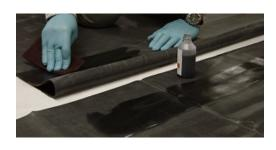
3. Add a small amount of the QuickPrime Plus onto the QuickScrubber Pad. Scrub this onto the two surfaces that are to be joined, ensuring there is a band of at least 100mm on each piece. On the bottom sheet this should go up to the drawn line and on the top up to the edge of the liner. Ensure the QuickPrime Plus is applied evenly, without streaks or puddling.
