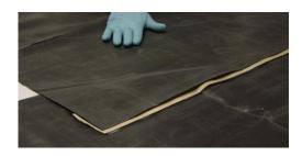
6. Do not peel off the backing of the QuickSeam Tape. Flap the top liner back over the bottom liner and line it up so that there is at least 6mm of the QuickSeam Tape backing paper visible.
