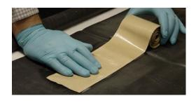
4. Lay one piece of the liner over the top of the other so that there is a minimum 100mm overlap. Mark a line on the bottom liner 10mm from the edge of the top liner.
