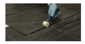
8. Use the Seam Roller to apply firm pressure firstly across then along the join length, including the edge, to ensure the whole join area is evenly bonded to both sides. Do not use your hands as the pressure will not be distributed evenly.
