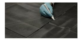
1. Lay one piece of the liner over the top of the other so that there is a minimum 100mm overlap. Mark a line on the bottom liner 10mm from the edge of the top liner.
