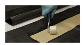
5. Use the Seam Roller to firmly press the QuickSeam Tape onto the bottom liner. This ensures there are no bubbles and that the Tape is evenly bonded to the liner. Do not use your hands as the pressure will not be distributed evenly.
