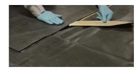
7. Carefully remove the backing paper from the QuickSeam Tape (it is best to do this by pulling it off at a 45-degree angle to the tape) whilst simultaneously pressing the top liner down onto the tape.
